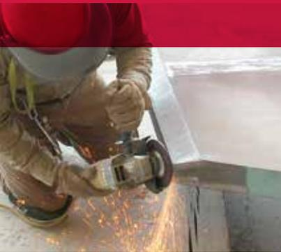
Grinding on a platform for weld preparation.
